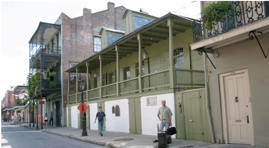
Figure 1. Madame John's Legacy, a 1789 brick and wood building in the French Quarter of New Orleans which is affected by soluble salts.
